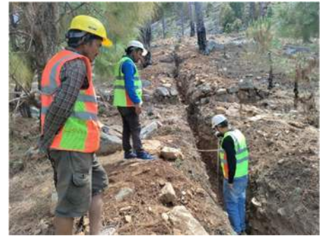
Photo 2: Inspection of environmental compliance and quality in Jukepani WSS,
