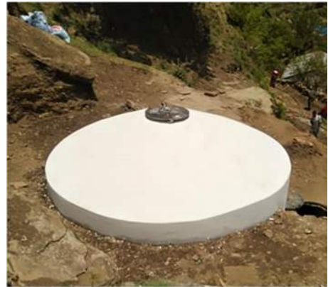
Photo 1: Complete RVT construction, Gorshekhola WSS
