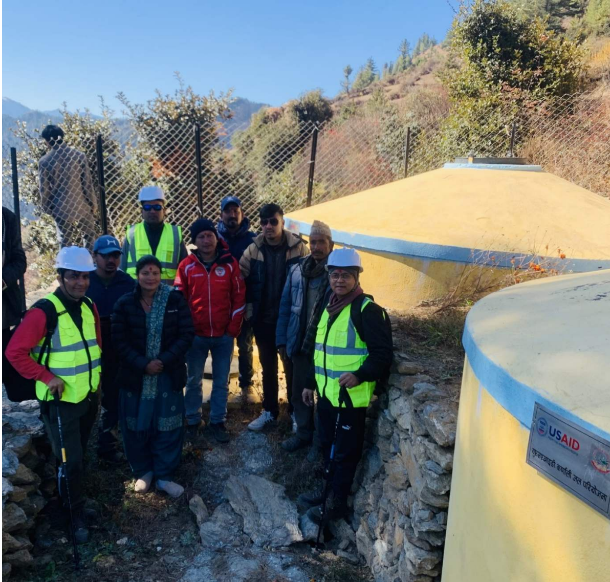
Photo: On November 23, 2023, the Nepal Engineering Services (NES) team, a third party, observed the implementation of the Murma Water Supply System (WSS) in Murma.
