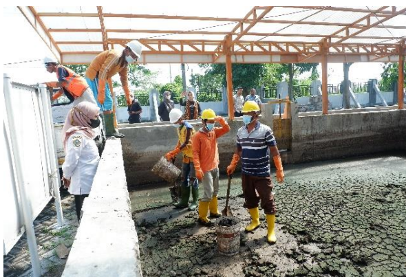
UPTD PLCD Gresik workers harvesting dry fecal sludge at the Betoयोगuci IPLT.
