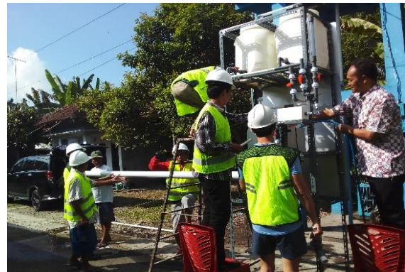
The pilot project of hydrodoser installation in the communal water supply system (SPAM) in RT3/RW6 in Kedungsari urban village, North Magelang sub-district, Magelang city. The installation takes place from May 23 rd to 25 th , 2023 and involves the communal SPAM caretaker group. W6.
