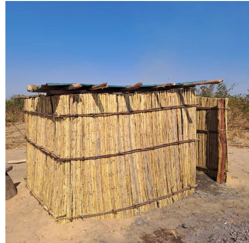
Photo Credit: [REDACTED]: Community members in Nalolo district constructing Baruto Model toilets.
