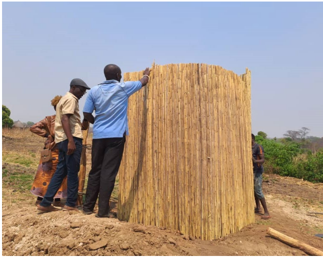
Photo Credit: [REDACTED]: Community members in Nalolo district constructing Baruto Model toilets.
