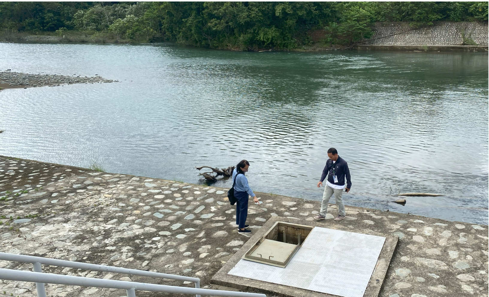
PUERTO PRINCESA CITY WATER DISTRICT RESERVOIR
