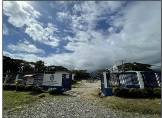
PPCWD- Montible Rive Intake Pumping Station
