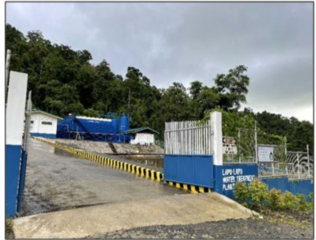
PPCWD Lapu-Lapu Water Treatment Plant
