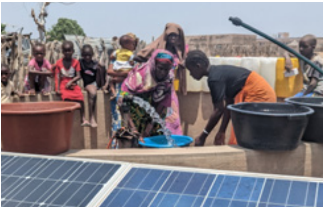
Solar-powered water pump in Sinthiou Mamadou Siré, Senegal. © Tetra Tech for USAID.
