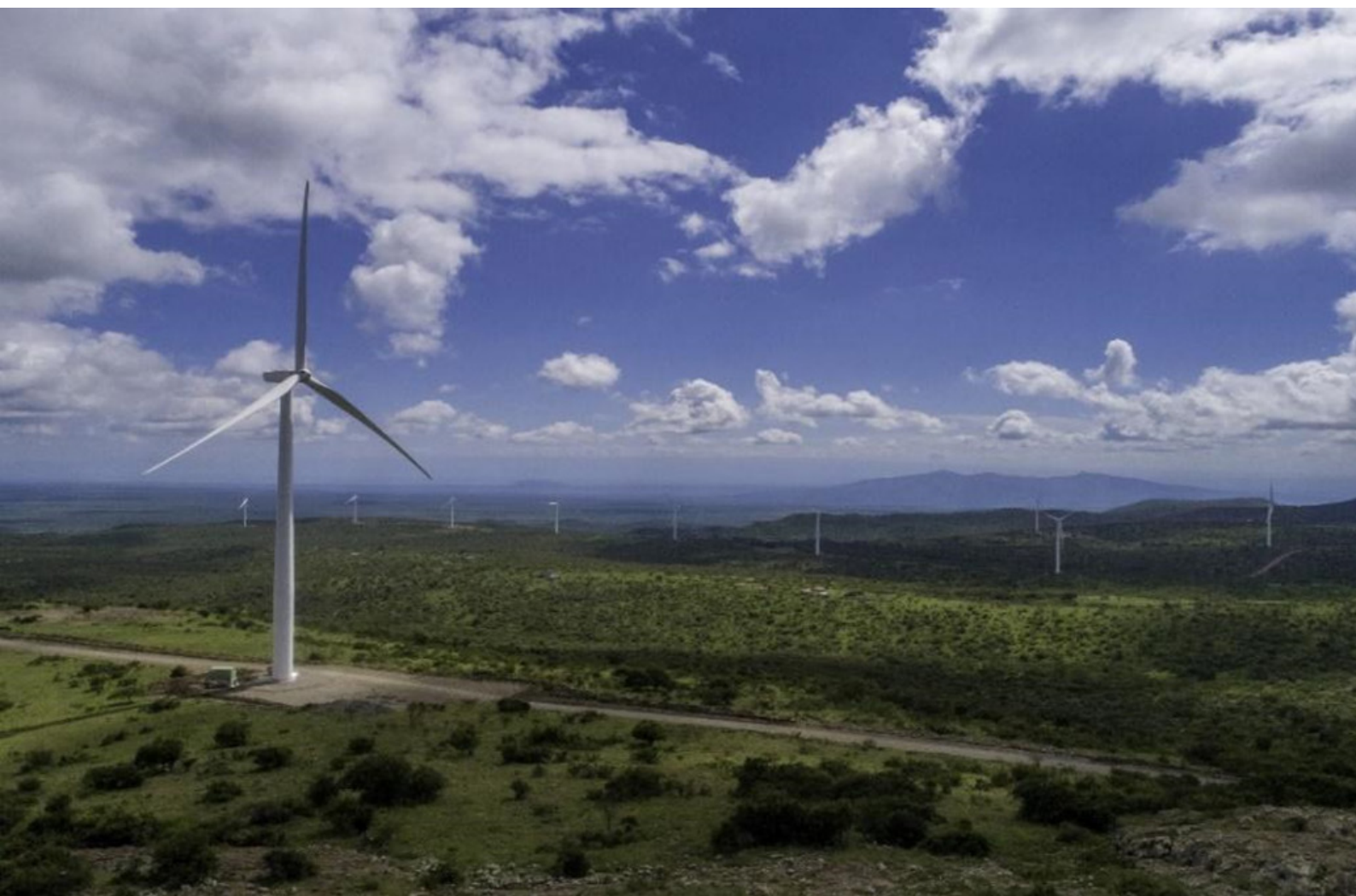
The 100 MW Kipeto Wind Farm power project. Photo credit: USAID/Kenya, Mwangi Kirubi
