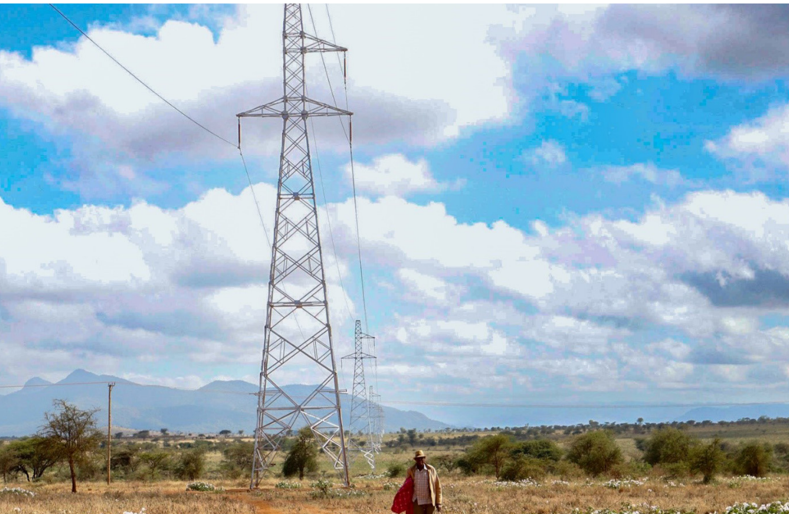
In Pako Village, Kenya, a man walks the wayleave or right-of-way of the Kenya Electricity Transmission Company Ltd. (KETRACO) towers of the 101 km Sultan Hamud–Oloitoktok transmission line project. Photo credit: EAEP
