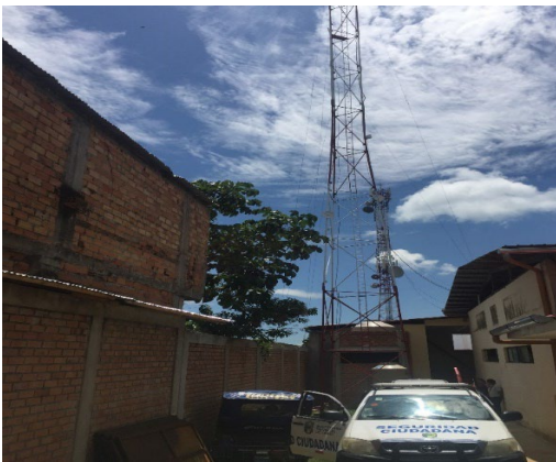
Lamas. Tower and water tanks
