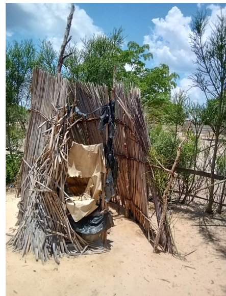
Traditional pit latrine susceptible to collapsing due to design failures in the substructure. Photo Credit: Costa Chitanda
