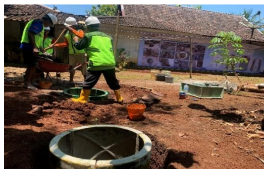
Training and Practice in Building SNI Standard Septic tanks included in the Negative Determination with condition (NDWC) category, wherein the training provides understanding of safety work and mitigation of potential dangerous activities.
