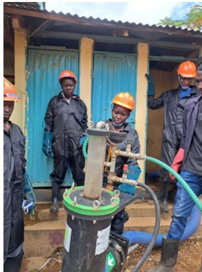
Exhibit 3. Pit emptiers from Changers Sanitation Group, led by Sheryl Achieng, during the Pupu pump training in Kisumu. Photo: USAID WKSP
