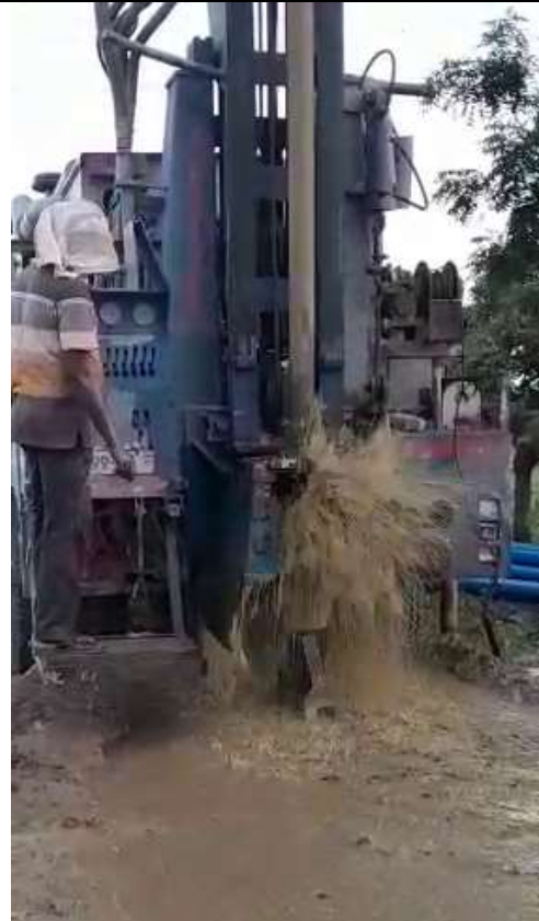
Drilling of borehole at Kpazie CHPs compound
