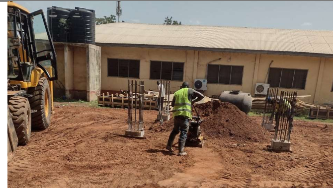
Compaction of foundation base at Tamale West Hospital
