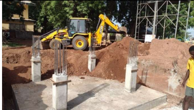
Construction of elevated tank starter columns
