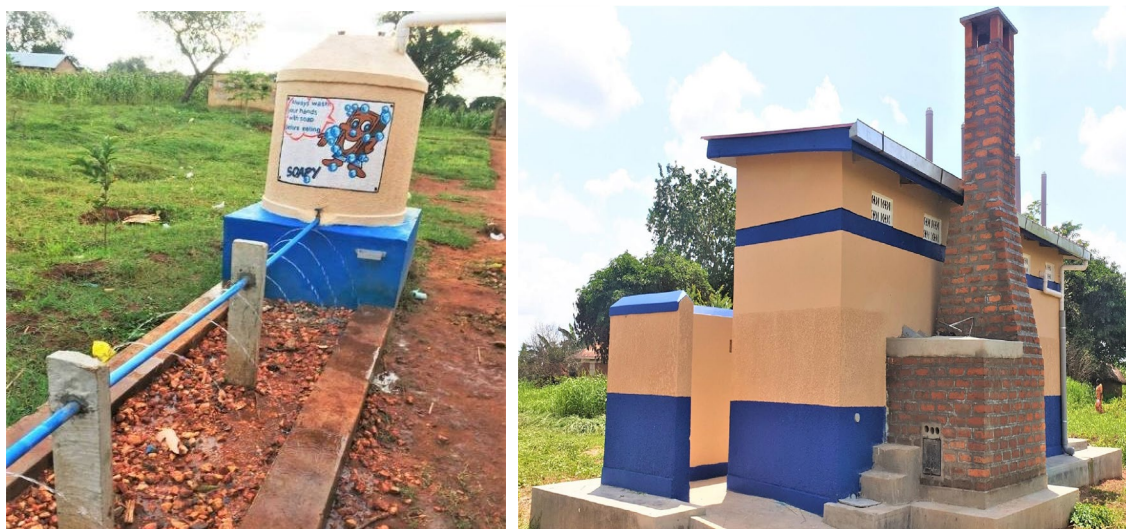
On the left, a group handwashing facility. On the right, an incinerator attached to girls’ toilet (Ikonia Primary School, Luuka district, Uganda)
