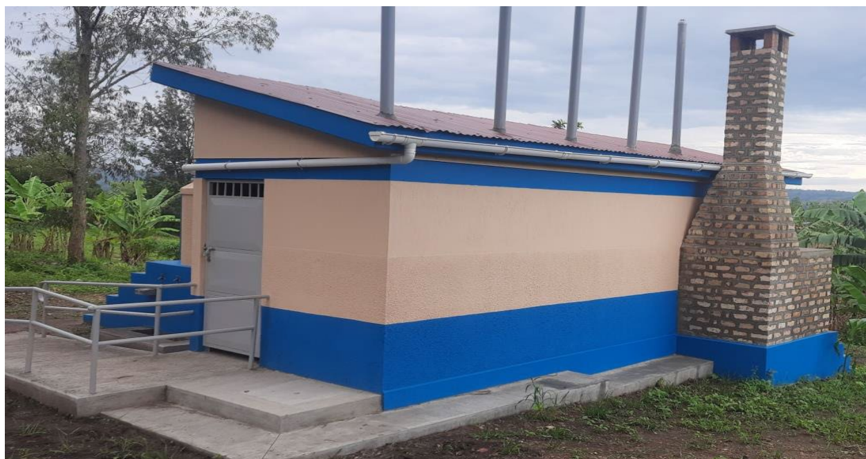
A newly constructed female-stance toilet with an MHM changing room and incinerator
