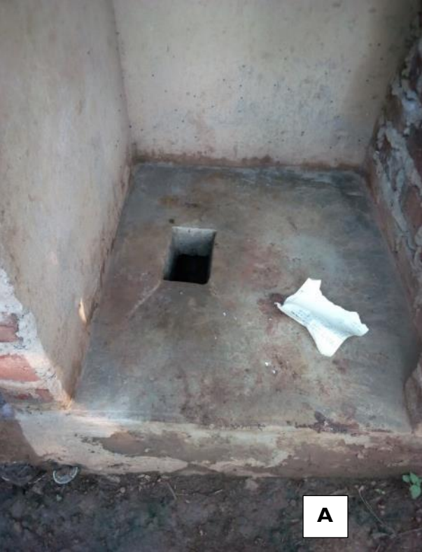
FIGURE 4.1. Examples of Latrines with Slabs (A and B) and without Slabs (C and D)
