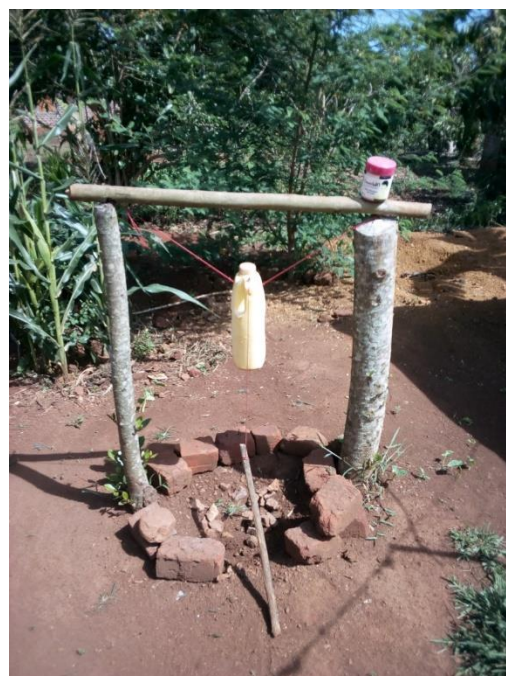
Figure 6.2: “Tippy Tap” Handwashing Facility within 10 Meters of the Toilet
