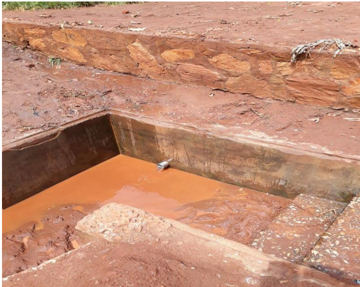
Figure 5.8: A Protected Spring in Buteme-A Parish, Buikwe District
