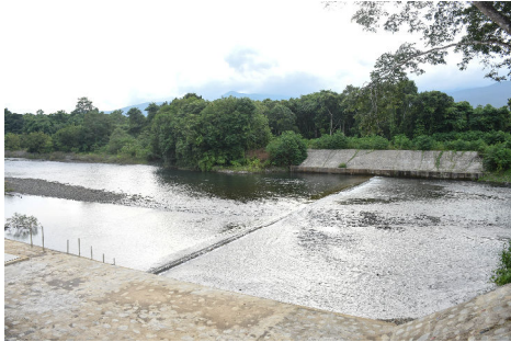
Sedimentation threatening water sources. USAID Safe Water team led by Chief of Party Alma Porciuncula joins PPCWD staff in inspecting sedimentation at the teruvian dam in Montible River. Bottom photo, courtesy to PPCWD.
