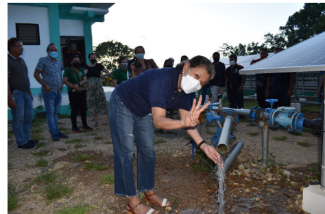
W is for Water. (Top) Mr. John Edgar, Environment Office Chief of USAID Philippines, joins participants to the three-day training on operations and management (O & M) of water supply facilities on April 21, 2022, as part of Earth Day celebrations in Coron. (Bottom) Ms. Alma Porciuncula, Chief of Party of USAID Safe Water, joins participants to the water supply operations and management (O & M) training during the site visit to Coron municipality's solar-powered deep well pump and chlorination system in Barangay Decalachao.
