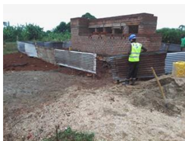
Figure B-1: Cordoned-off Construction Site
