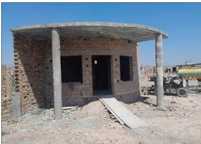
Photo 05: Guard room structure completed.
