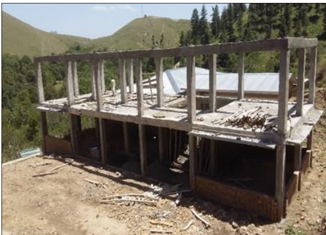
Photo 05: Construction view of main school building – GPS Kool, Orakzai
