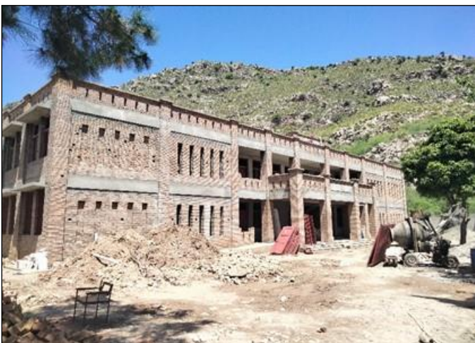
Photo 11: Construction view of main school building – GGMS Suni Khel, FR Kohat
