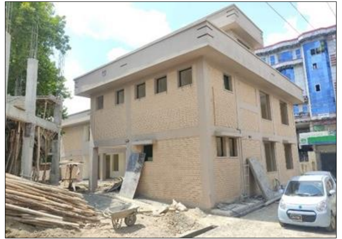
Photo 15. Construction view of Line Department Offices building – Tehsil-Level Government Complex, Swat
