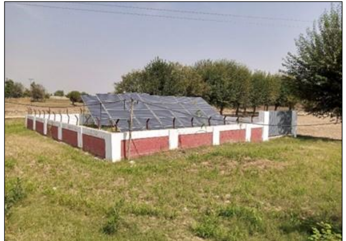
Photo 04: Solar panel compound completed – DWSS Loe Jowar Khar, Bajaur
