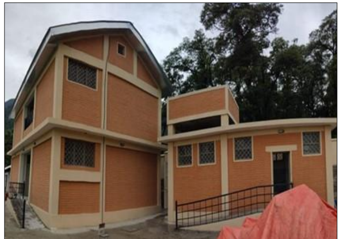
Photo 06: Construction view of Module T-7 and lavatory block – GPS Talkar, Swat
