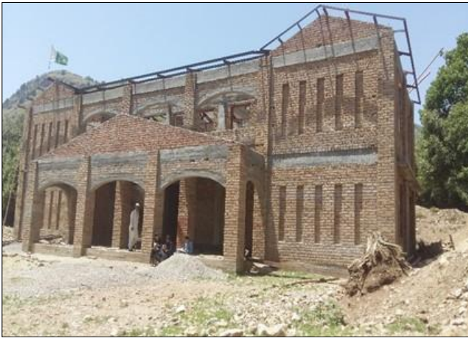
Photo 09: Construction view of main school building – GPS Garhi Mishti, Orakzai
