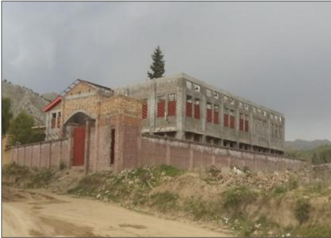
Photo 01: Construction view of project site – GGHS Togha Sam, Orakzai
