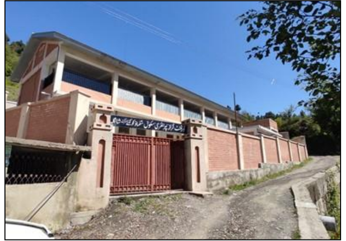
Photo 13. Construction view of project site – GGPS Shalmano Kotkay, Shangla
