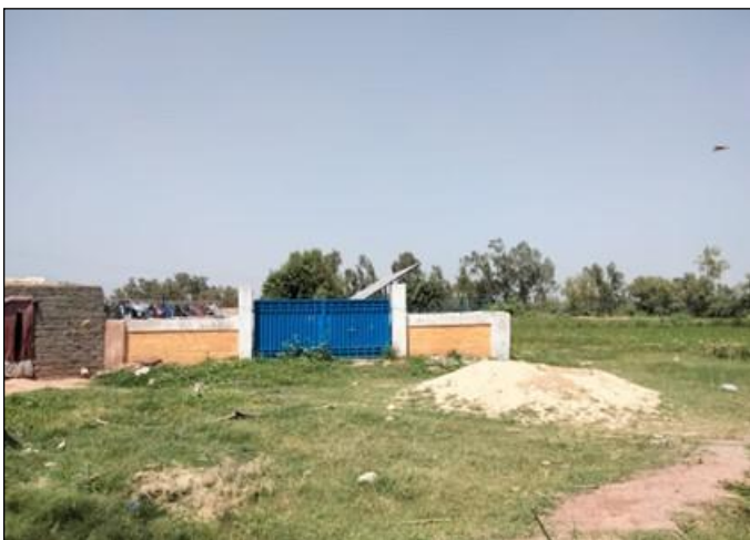
Photo 11: Solar panel compound completed – IWSS TW#07 Toheed Abad, Khyber
