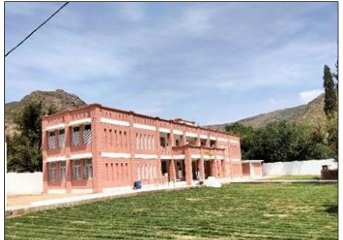
Photo 04: Construction view of main school building – GGMS Jammu Shahi Khel, FR Kohat
