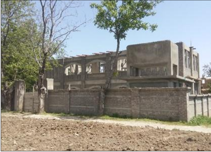
Photo 07: Construction view of project site – GGPS Zanka Khel, Orakzai
