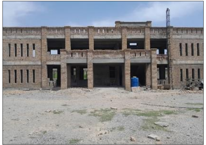
Photo 10: Construction view of main school building – GGPS Janat Khan, FR Peshawar
