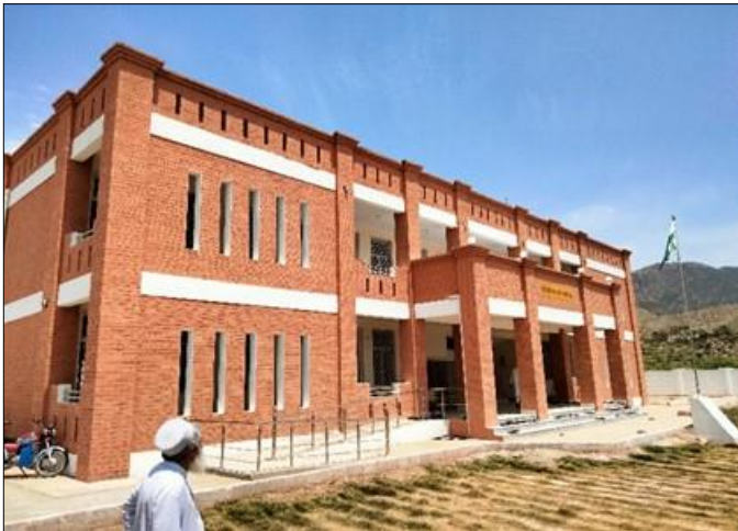
Photo 03: Construction view of main school building – GPS Shahi Khel, FR Kohat
