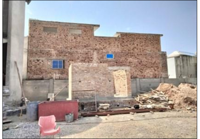
Photo 02 Brick work of fire pumping system partially completed.
