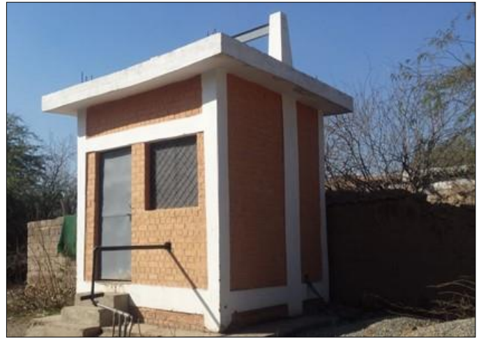
Photo 02: Pump house completed – DWSS Ghundi 5 Jamrud, Khyber
