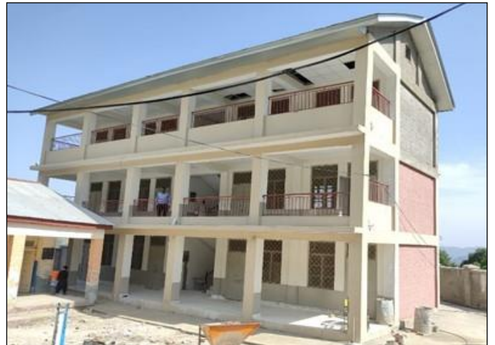
Photo 04: Construction view of Module T-13 – GPS Dardyal, Swat
