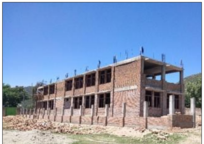
Photo 12: Construction view of main school building – GGMS Bilal Kalay, FR Kohat
