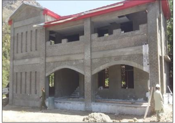
Photo 08: Construction view of main school building – GGPS Dago Takhtak, Orakzai
