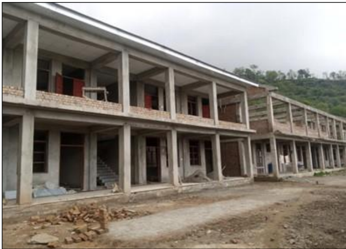
Photo 14. Construction view of Module T-4 and T-6 – GHS Mirgambala, Dir Lower
