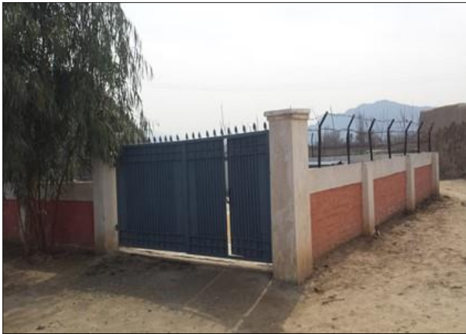
Photo 09: Solar panel compound completed – IWSS Gul Zada, Mohmand
