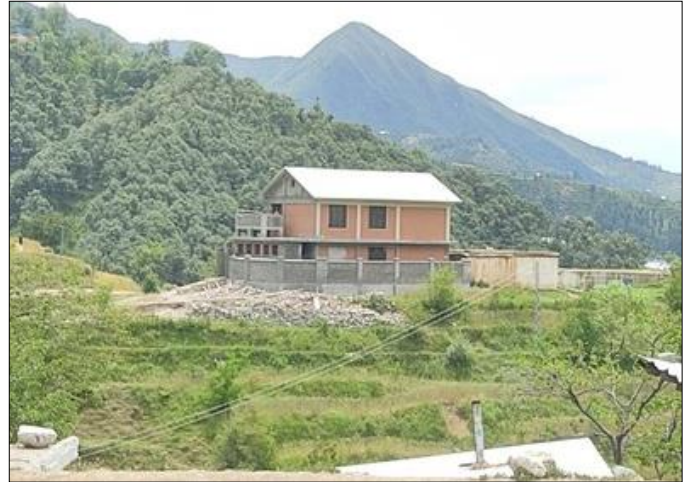
Photo 02: Construction view of project site – GPS Bahadar Banda, Swat
