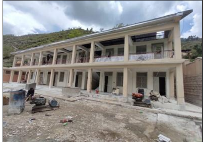
Photo 08: Construction view of project site – GPS Shomnai, Dir Upper
