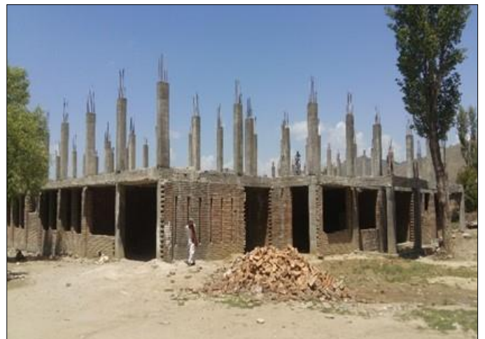
Photo 06: Construction view of main school building – GHS Awi Mela, Orakzai
