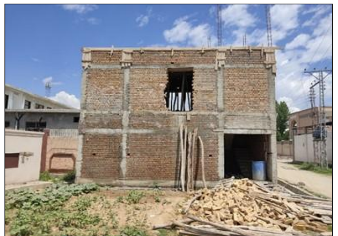
Photo 17. Construction view of servant quarter No. 1 – Tehsil-Level Government Complex, Swat
