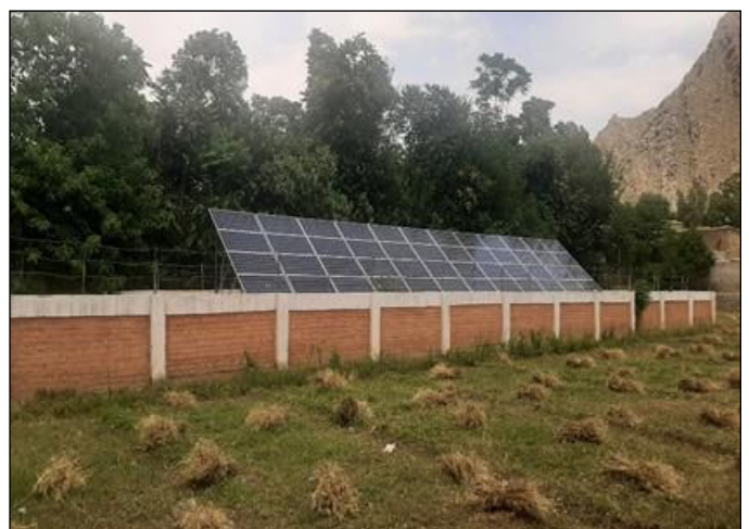
Photo 06: Solar panel compound completed – IWSS 31/ 2046 Safi I, Mohmand
