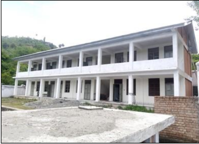
Photo 12. Construction view of Module T-3 – GPS Loyal Namal, Swat
