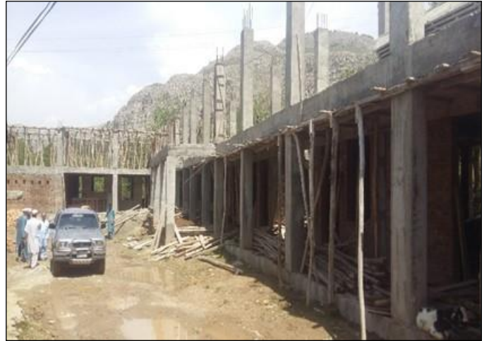
Photo 02 Construction view of main school building – GGHS Spen Beghi, Orakzai
