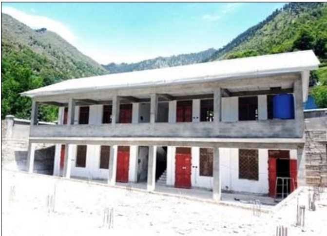
Photo 03: Construction view of Module T-4 – GGPS Kalagay, Swat
