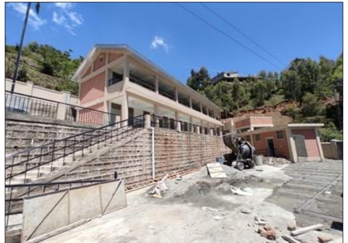
Photo 10: Construction view of Module T-3 and lavatory block – GPS Mailaga, Swat
