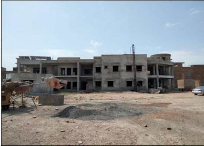
Photo 01: Front view of main administration building.
