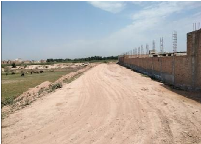
Photo 03: Subgrade of the road along boundary wall completed.
