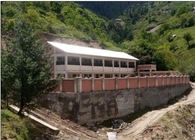
Photo 09: Construction view of project site – GPS Fatima, Swat
