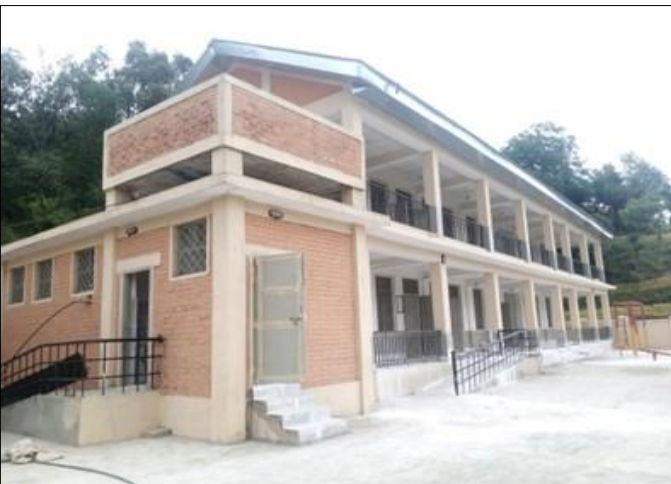
Photo 05: Construction view of Module T-3 and Lavatory Block – GPS Pansat, Swat
