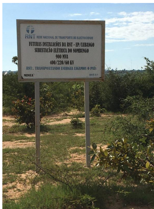
New Lubango substation construction site. Photo: SAEP
