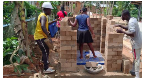
Latrine artisans training on superstructure for HHLs
