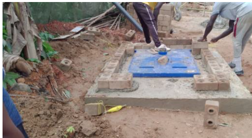
Latrine artisans training on Digni-Loo installation
