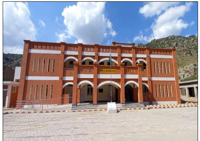
Photo 04: Front view of main school building – GGPS Zoor Kalay, FR Kohat
