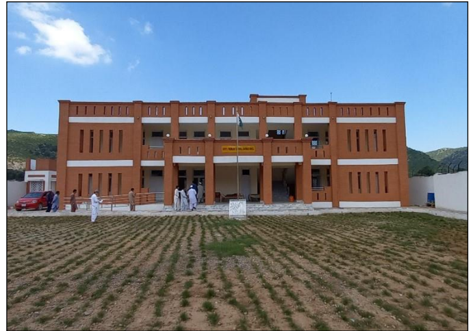
Photo 02: Front view of main school building – GPS Sarwar Khel, FR Kohat
