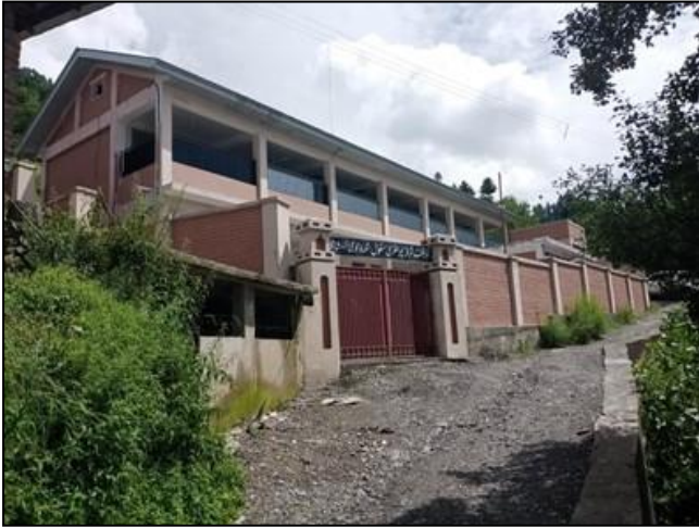
Photo 12. Construction view of project site – GGPS Shalmano Kotkay, Shangla
