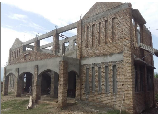
Photo 05: Construction view of main school building – GPS Kasim Khel, Orakzai
