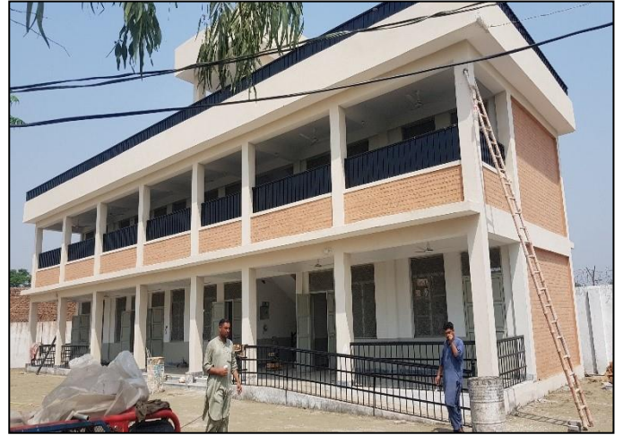
Photo 13. Construction view of Module M-3 – GPS Karam Khel Mushtarzai, Peshawar
