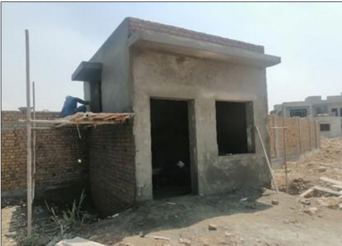
Photo 03: Plastering and backfilling of electric room in progress.
