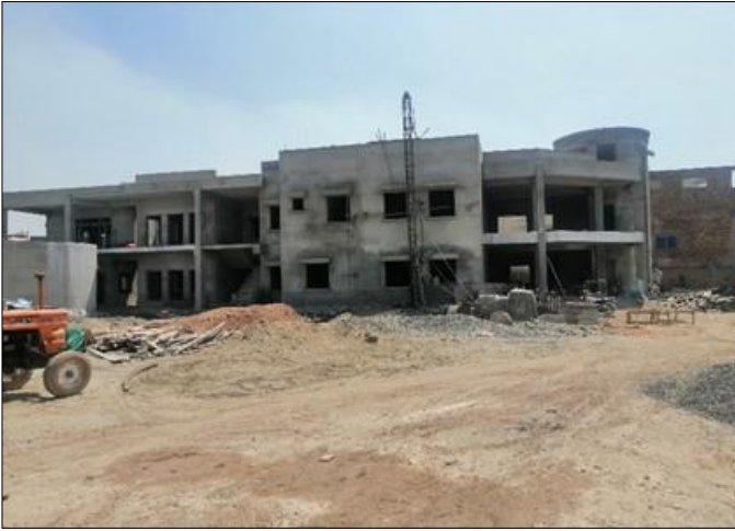
Photo 01: Front view of Administration Building.
