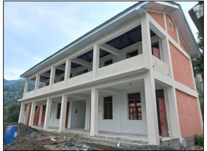
Photo 08: Construction view of Module T-4 – GPS Qala Qalagai, Swat
