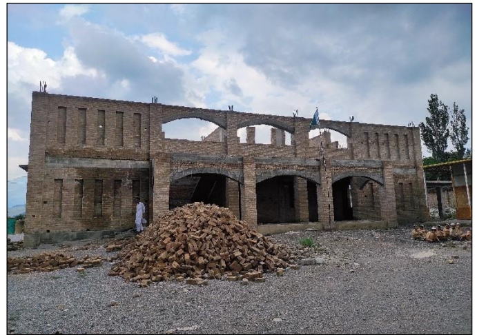
Photo 08: Construction view of main school building – GPS Star Jumat, Kurram
