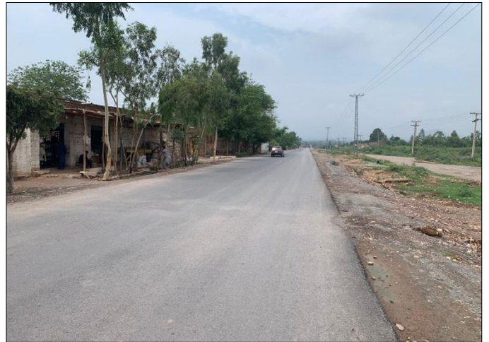
Photo 02: Asphalt wearing course completed from RD 0+000 to RD 5+000 – Bara to Mastak Road, Khyber
