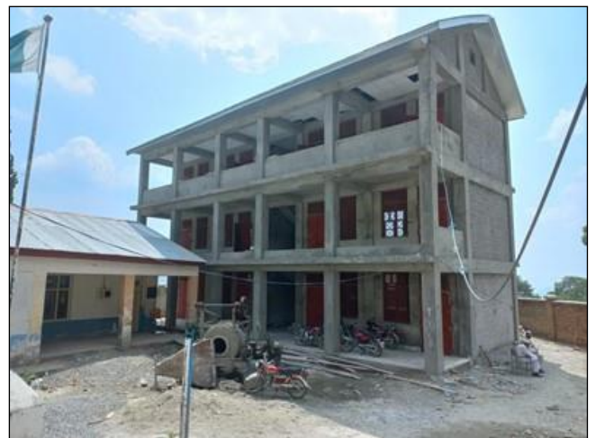
Photo 17. Construction view of Module T-13 – GPS Dardyal, Swat
