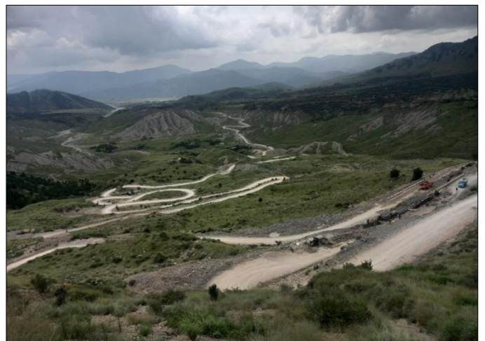
Photo 06: Overview of road – Ghiljo to Dabori Road, Orakzai
