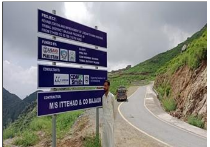
Photo 04: Diamond grade sheet fixed on project board at RD 23+775 – Loesam Nawa Pass Road, Bajaur
