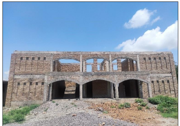
Photo 12: Construction view of main school building – GGPS Maro Khel, Kurram
