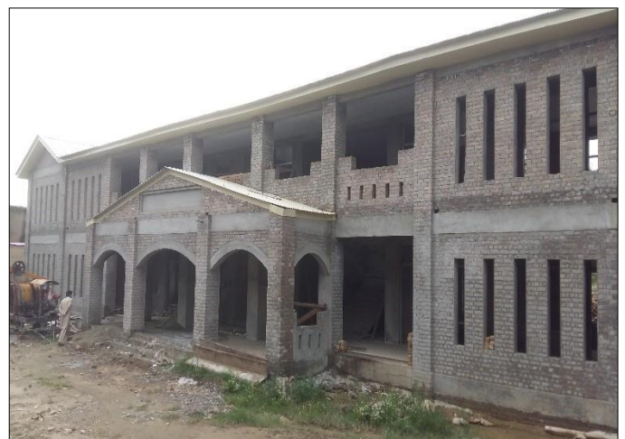
Photo 06: Construction view of main school building – GGMS Tooti Bagh, Orakzai
