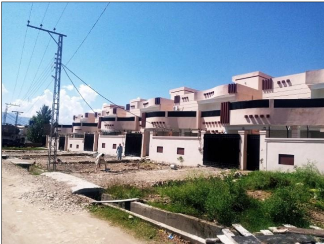
Photo 01: Status of works at Residences No 1 to 5 – Tehsil Level Complex, Swat
