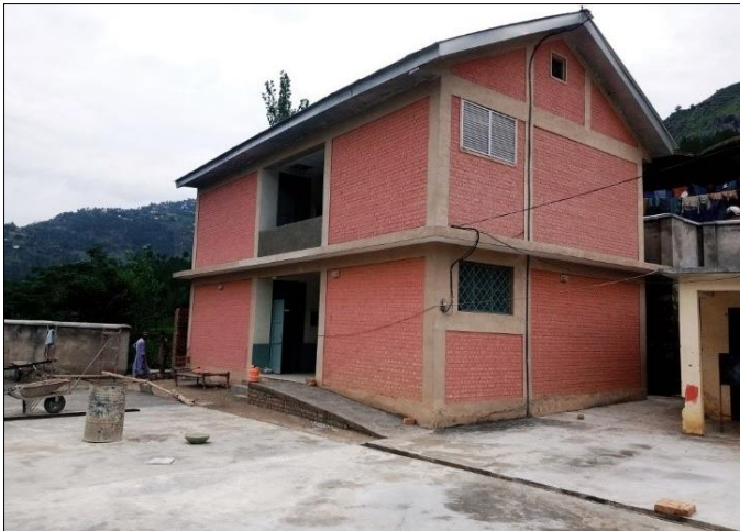
Photo 03: Construction view of Module T-7 – GGPS Look Maira, Swat
