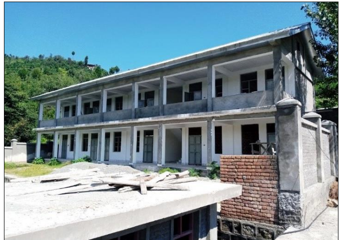
Photo 02: Construction view of Module T-3 – GPS Loye Namal, Swat
