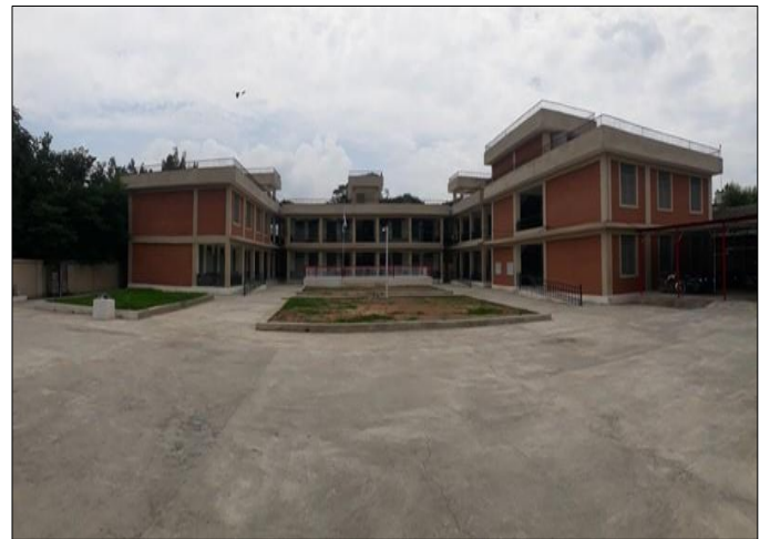
Photo 15. Construction view of project site – GHS Mian Brangola, Dir Lower
