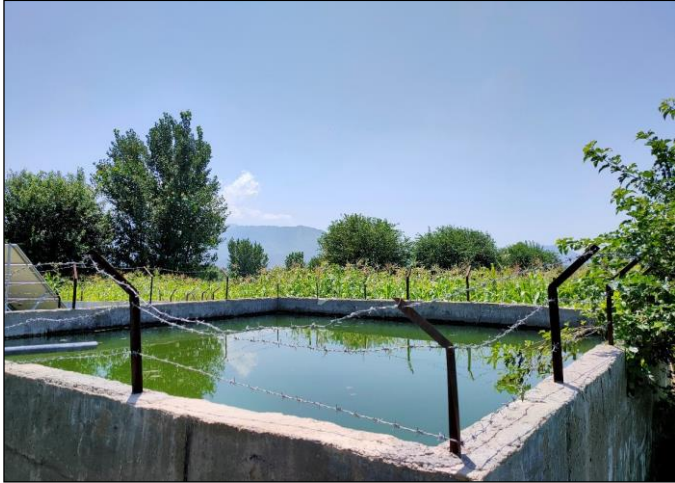
Photo 07 Surface water tank constructed at site – IWSS Mulano Killi, Bajaur
