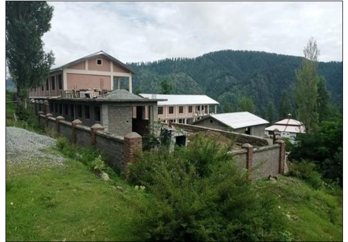
Photo 10: Construction view of project site – GHS Amnavi, Shangla
