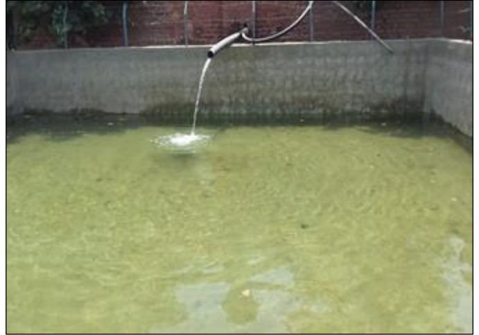
Photo 08 Surface water tank is operational – IWSS SK-2 Shahkass 2, Khyber
