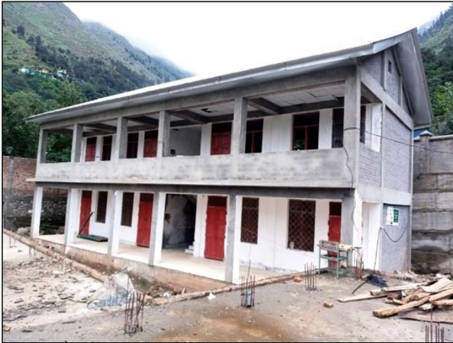
Photo 09: Construction view of Module T-4 – GGPS Kalagay, Swat
