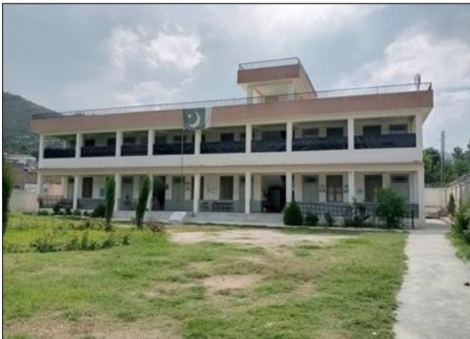
Photo 14. Construction view of Module M-1 – GPS Hisar Baba, Malakand
