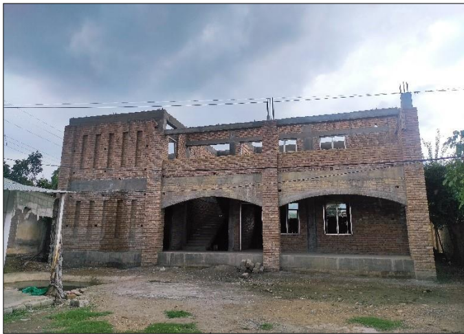
Photo 07: Construction view of main school building – GGPS Khurmana, Kurram
