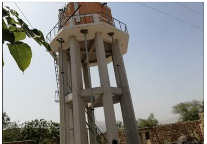
Photo 04: Overhead water tank completed at site – DWSS Shahkass 3 Jamrud, Khyber
