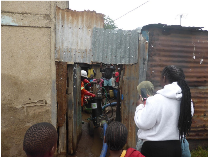
Exhibit 2. USAID WKSP project staff assessing the Ghasia Poa FSM group using the mechanized pit-emptying process using Pupu Pump in Manyatta informal settlement in Kisumu County. Photo: USAID WKSP
