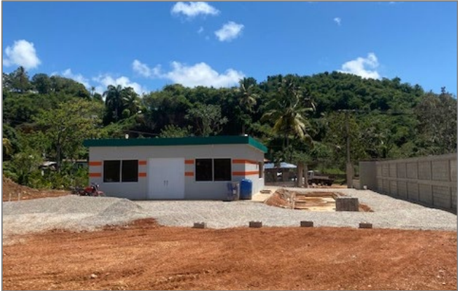
New facilities and fencing installed at the Santa Barbara landfill site. Source: Sostenibilidad 3Rs for Clean Cities, Blue Ocean
