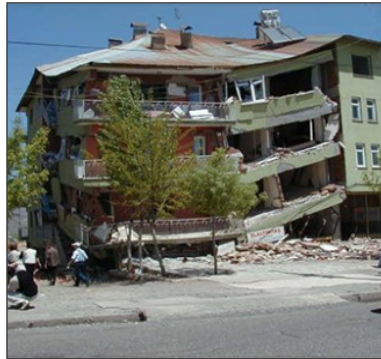
Residential Structure in Bingöl, Turkey (Photograph Credit B. Yön et al. )
