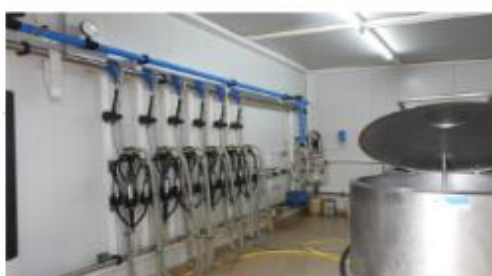
Milk Cooling Tanks
