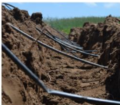
Subsurface drip irrigation system
