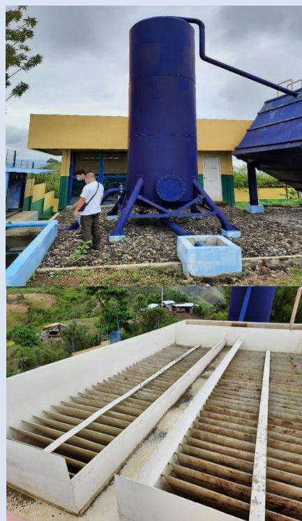
Above: Inspection of Flocculation Tank Below: Existing Plate Clarifier
