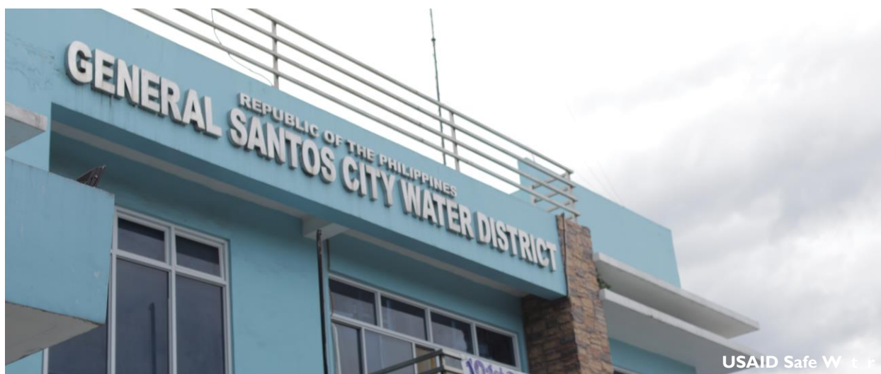
The USAID Safe Water team is engaging with the General Santos City Water District stakeholders in two of its development projects on surface water bulk supply development and the septage management program.
