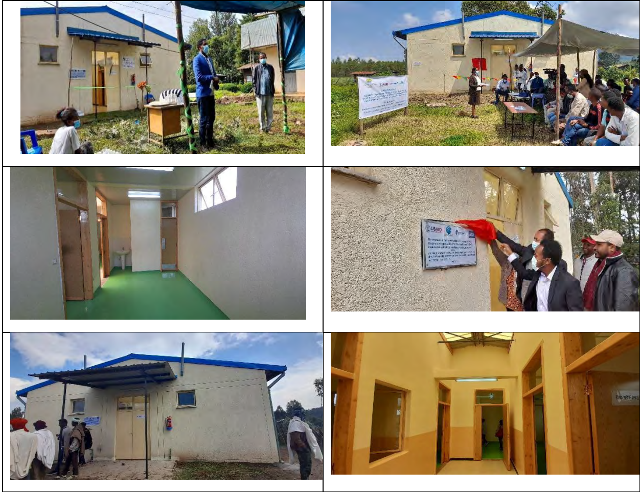
Photo 3,4,5,6,7 & 8: The completed renovation work of health facilities being handed over to the WorHOs in Amhara region (Durbete, Kidamaja, Maynet & Nefas Mewcha HCs)
