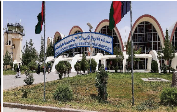
Photo #20: A-012-06_KDH site visit, Kandahar Province. MF, 2021-05-10.
