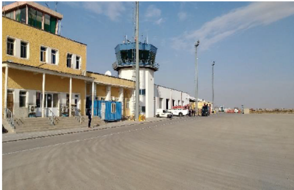
Photo #13: A-012-02 Site visit of the Mazar Airport, Balkh Province. MA, 2021-02-08.
