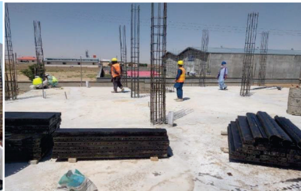
Photo #20: A-021_Office columns steel winding, Balkh Province. ZA. 2021-06-23.
