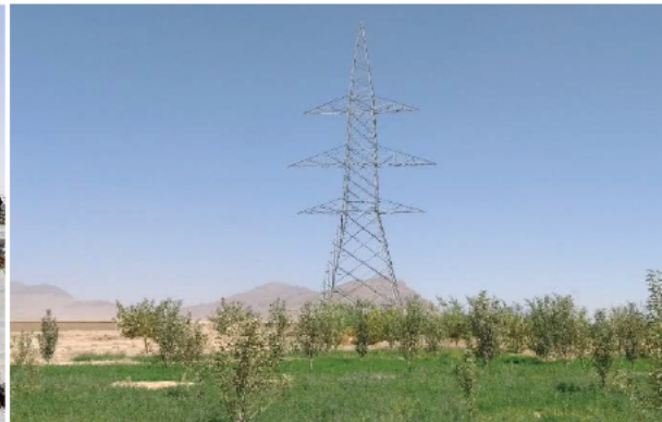
Photo #2: A-005_Structure erection at Tower No. MS 10-01, Ghazni Province. SS, 2021-09-21.
