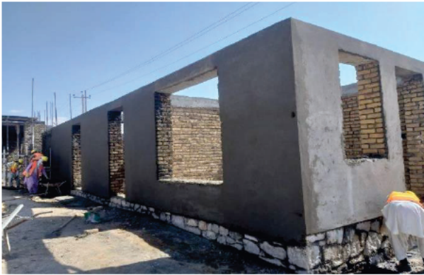
Photo #19: A-021_Cloak and guard room plastering, Balkh Province. ZA, 2021-05-26.
