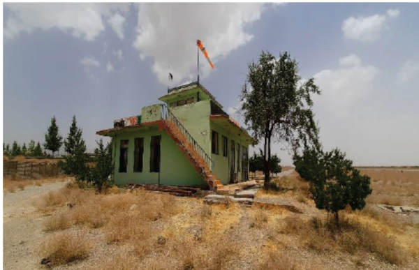
Photo #15: A-012-03 View of the control tower at the Gardez Airport, Paktya Province. MH, 2021-07-12.
