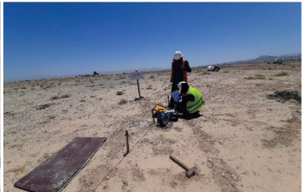
Photo #22: A-023_Digging test pit, Herat International Airport, Herat. MD, 2021-06-03.
