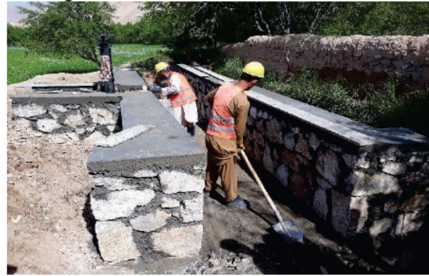
Photo #9: A-007_Turnout #13 cleaning, Qushpara Canal, Samangan Province. MY, 2021-04-11.
