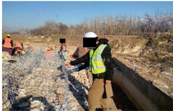
Photo #21: A-013_ Inspection of gabion works, Choghai Canal, Samangan Province. MHM, 2020-12-16.
