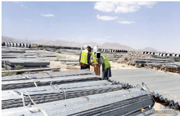
Photo #1: A-005_Materials inspection at Gelan Store, Ghazni Province. MK, 2021-07-01.
