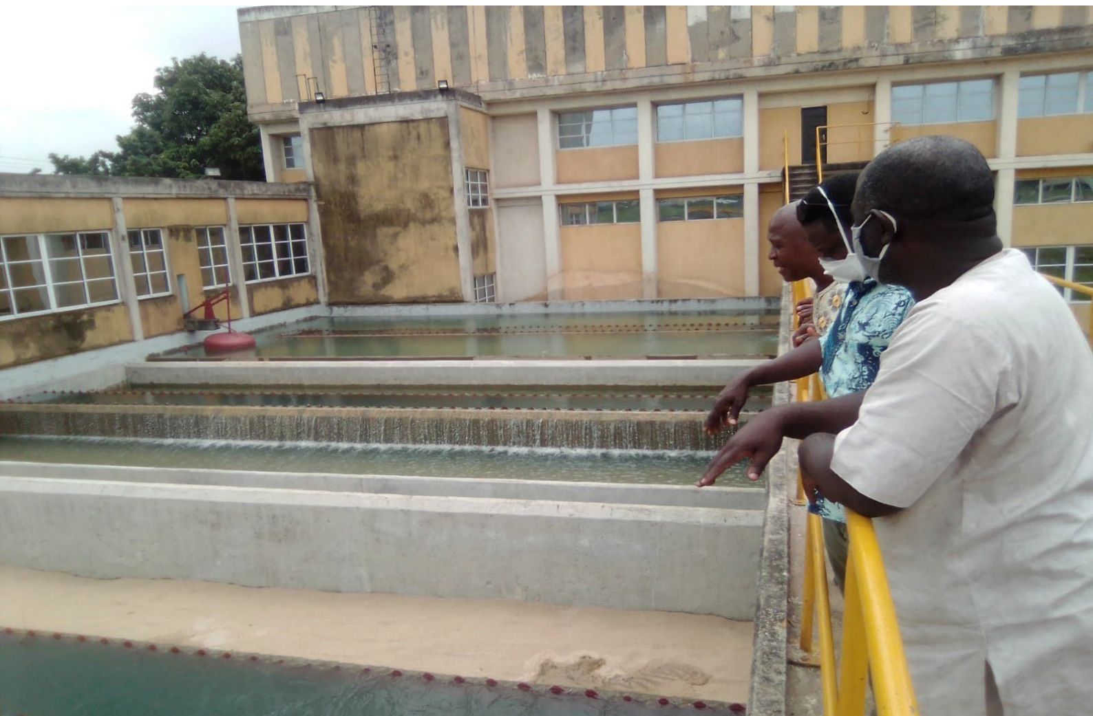
Filtration system at Otamiri Water Scheme/Treatment Plant, Owerri, Imo State (Photo credit: Engr. Tony Offor; August 18, 2020).
