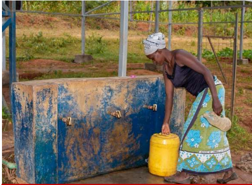
A lady fetches water from a communal point operated by a rural based Kanoto Water Project in Makueni County. KIWASH supported the project through installation of solar panels to reduce the pumping costs and constructed water distribution to increase water access.
