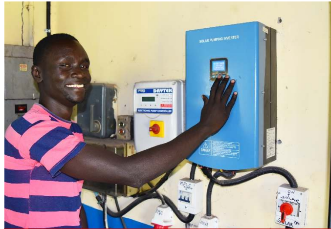
A water attendant operating a solar inverter installed by KIWASH for Nyang'oma Water Project in Kisumu County. KIWASH supported 22 WASH enterprises to install hybrid solar panels as a means of cutting operational costs and enhancing sustainability.
