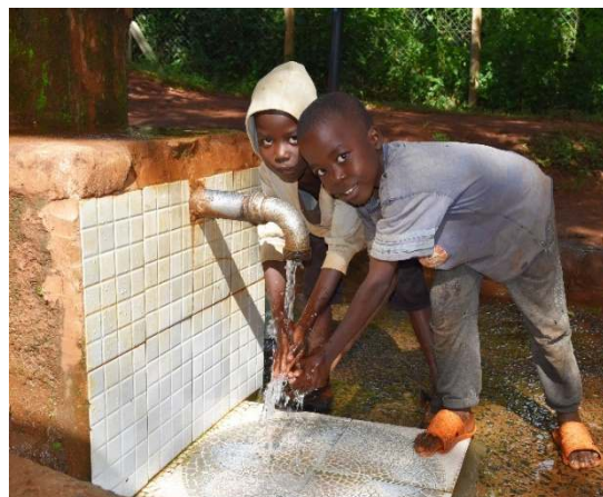
A KIWASH protected spring at Khwisero area in Kakamega County. Protection involved; construction of concrete spring boxes, fencing of local sources, construction of washing bays and cattle watering points and construction of a drainage channels to prevent water stagnation
