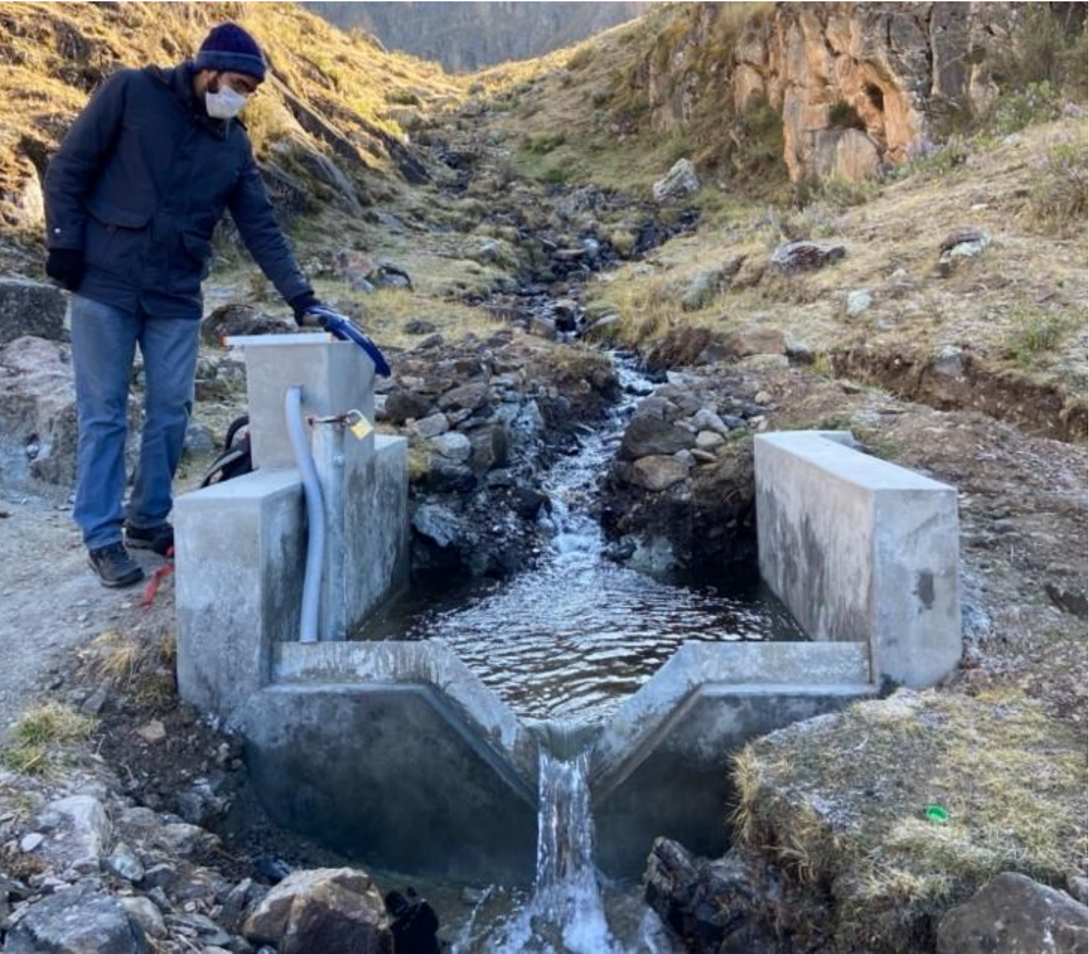
Project personnel are monitoring the operation of a weir in the upper Lurin river basin, Lima, Peru. This small construction for flow measurement is part of a network of rain gauges and various water level and temperature sensors to improve knowledge and decision making in the area. (Photography: CONDESAN).
