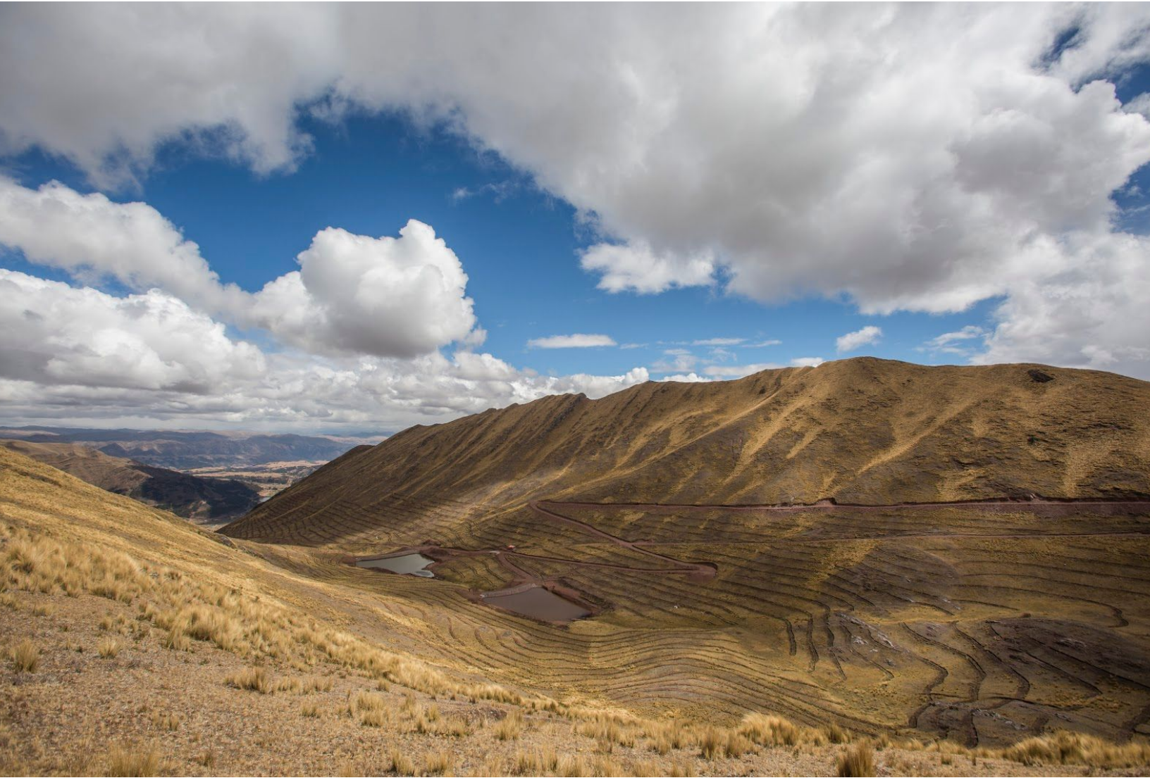
Infiltration trenches in Piuray, Cusco, helps the local population to have good quality and quantity of water to maintain their livelihood. (Photography: Forest Trends)
