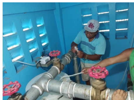
Officers of Purok Tres Lanton RWSA installed chlorinator after the visit of the SURGE Team.
