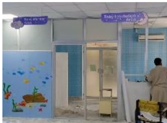
Photo1: Children ward under construction in City Hospital, Lakki Marwat
