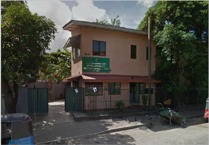
Figure 12. Solid Waste Management Depot CMC (Google Street View 11-2015)
