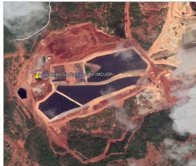
Figure 22. Aruwakkalu Sanitary Landfill (MCUDP) (Google Aerial 3-2020)
