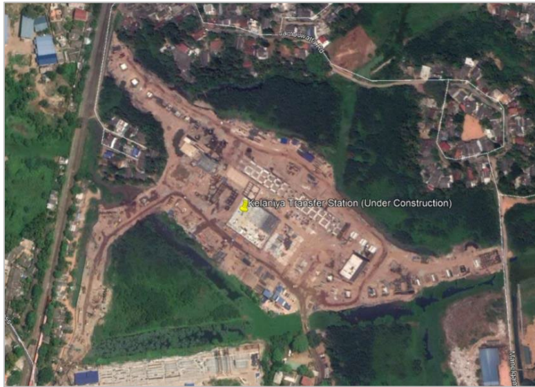
Figure 21. Kelaniya Transfer Station/Intermodal Facility (under construction) (Google Aerial 3-2020)
