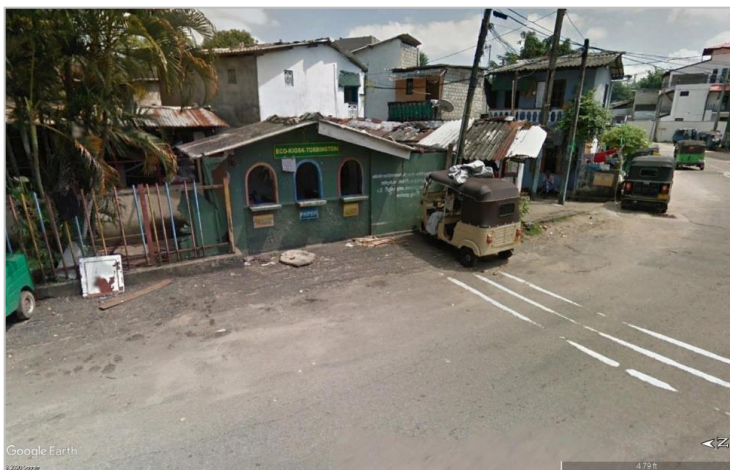
Figure 13. Eco-Kiosk Torrington (Google Street View 11-2015)
