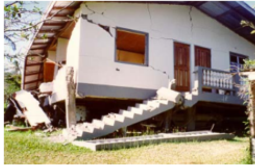
Figure 1 Tobago Earthquake Damage. Photo from uwiseismic.com
