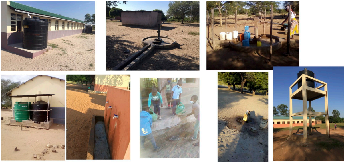
Figure 52: Photos of observed water infrastructure
