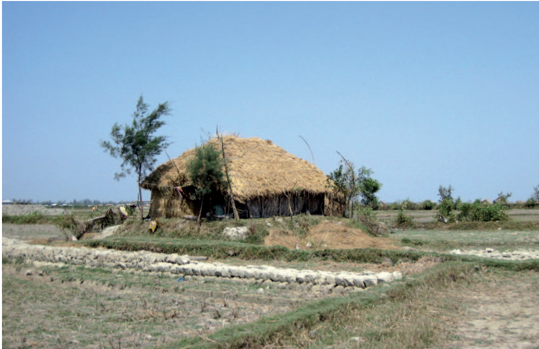
For flood protection, houses are constructed on an earth mound. © Judith Rosendahl
