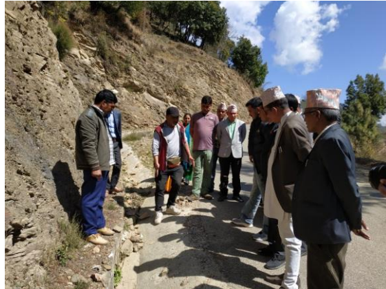
SWN rural road expert demonstrating how proper road geometry and a water drainage system help to make a rural road durable throughout the year. Photo credit: SWN
