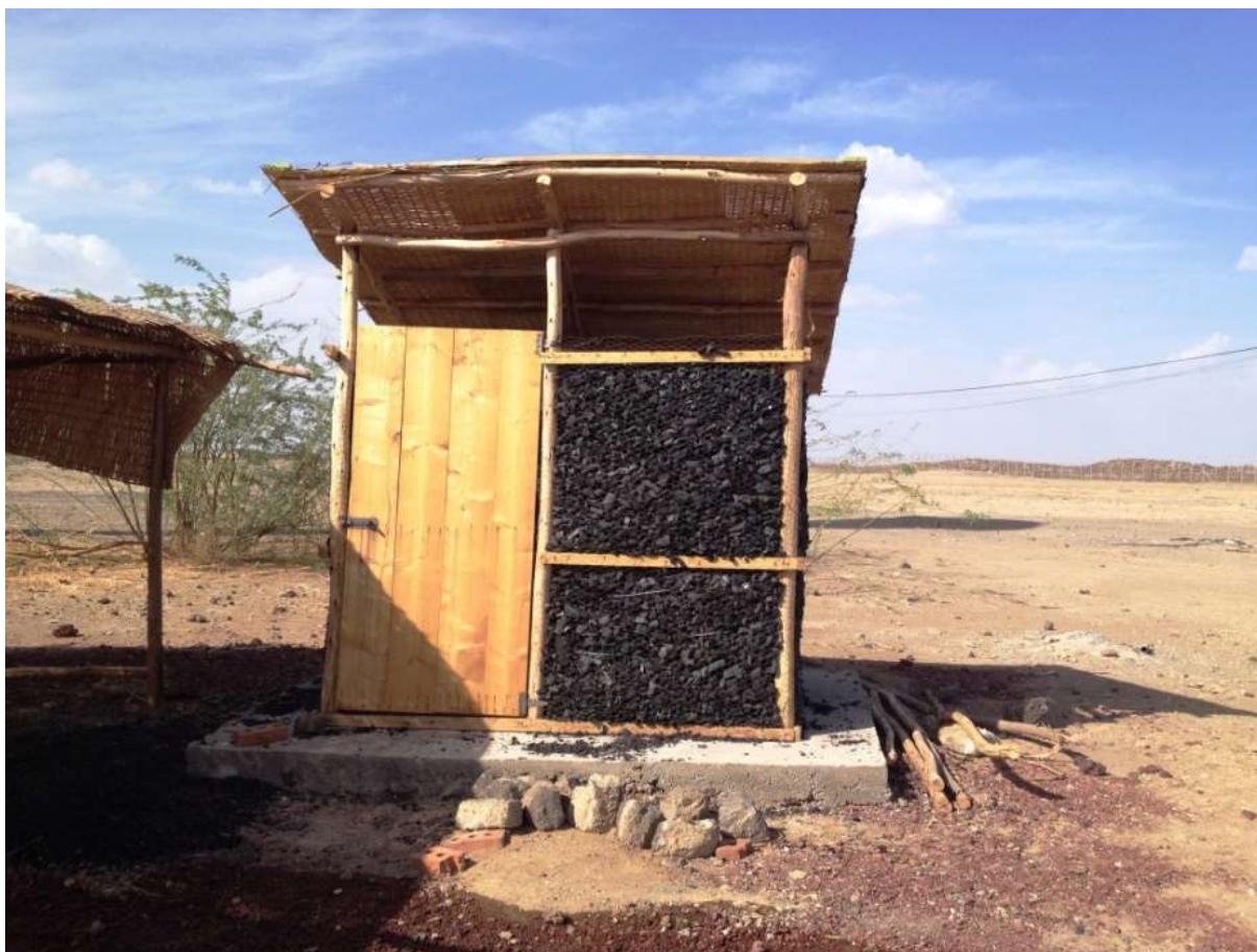
Figure 4: Walk-in size charcoal cool room for small-scale cool storage in Semera, Ethiopia. (Source: Lisa Kitinoja).
