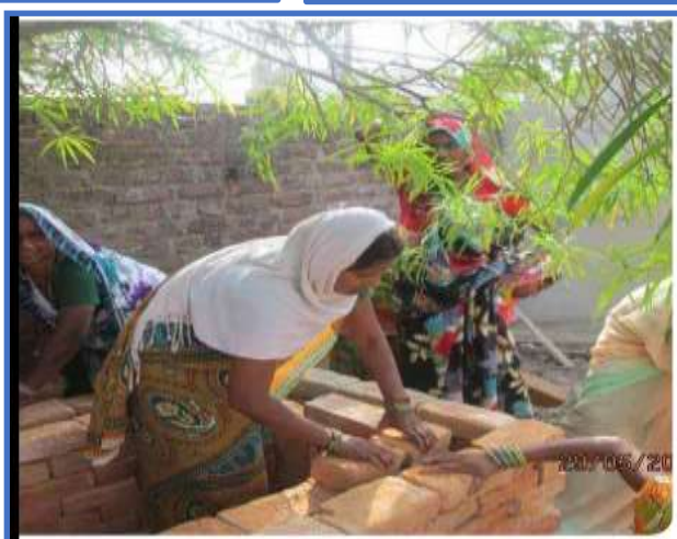
Upper Left: On-farm cellar storage managed by cooperatives; Upper Right: Low-cost shade structure, made using indigenous materials; Lower Center: Zero Energy Cool Chamber made with bricks and sand (Source: Padam Bahadur Subedi, Jumla, Nepal).
