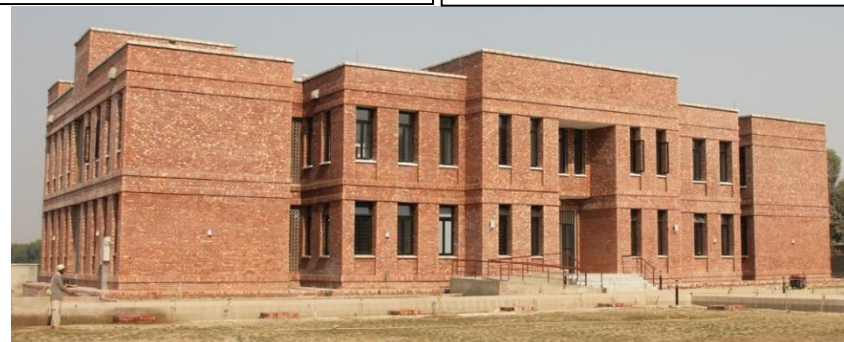
USAID Funded state-of-the-art school
