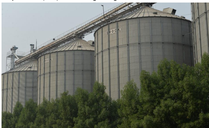
Grain storage silos
