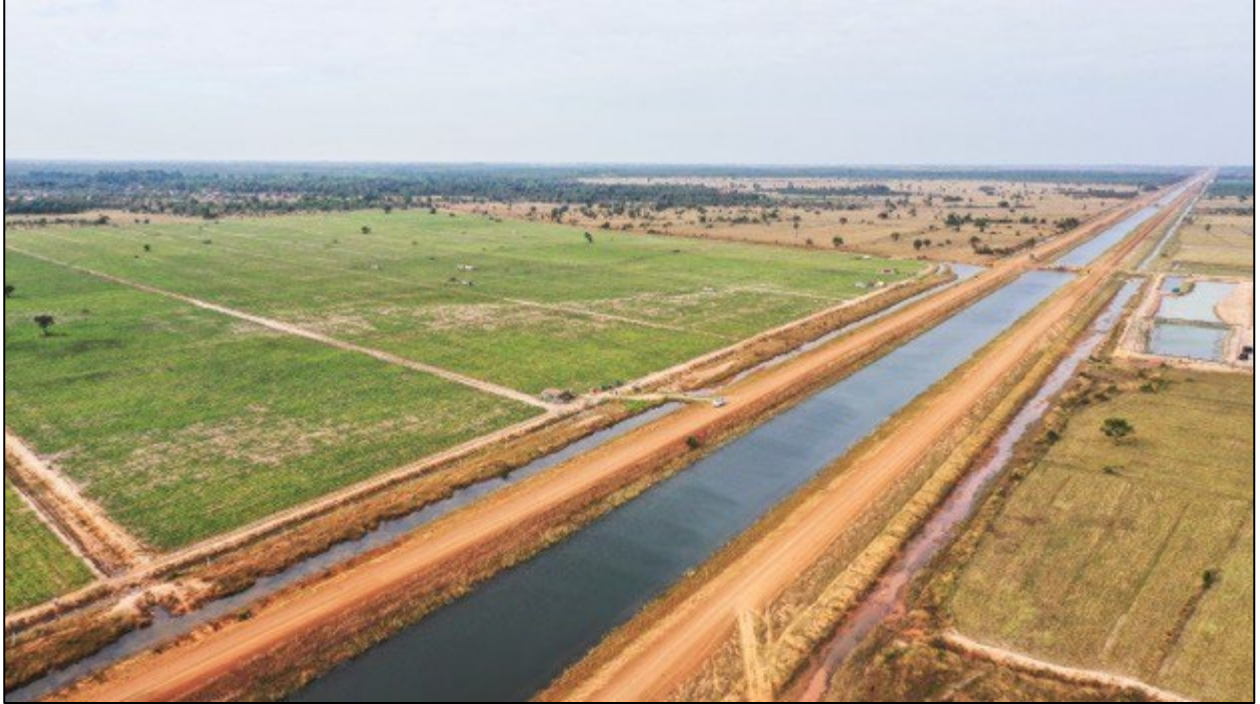
Visual Stories Photo 12: The Tang Krasang irrigation system main canal is about 30 km long and supplies water to many other canals, streams, and ponds over 10,000 ha of farmland.
