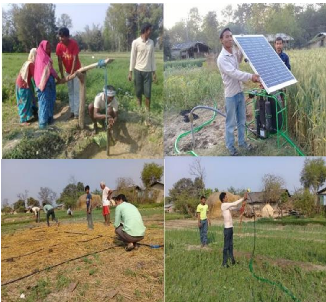
Figure 5-12: Micro irrigation technology and solar pump installation at Kuti village.
