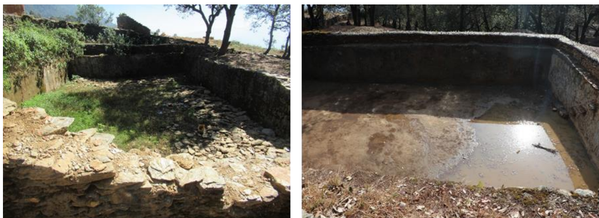
Figure 5-7: Raniban Pond, Mellekh village a) before intervention b) after intervention.
