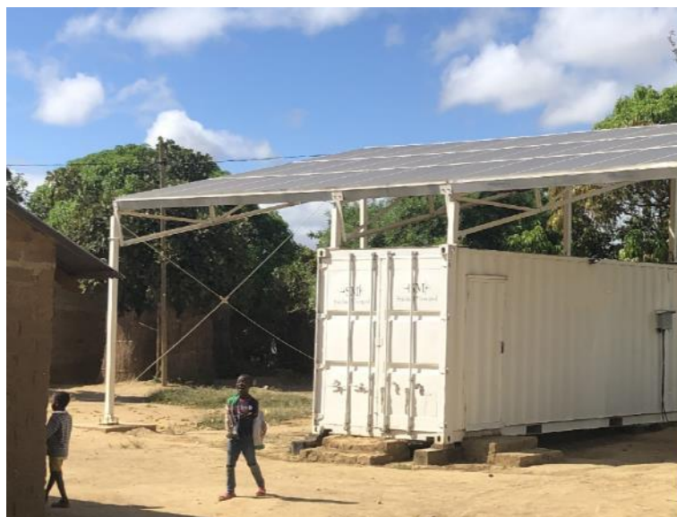
Figure 10: A mini-grid is an off-grid electricity distribution network involving small-scale electricity generation. Photo credit: USAID SAEP
