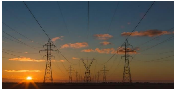
Building and maintaining reliable transmission infrastructure is crucial for increased electricity access. Photo Credit: RNT
