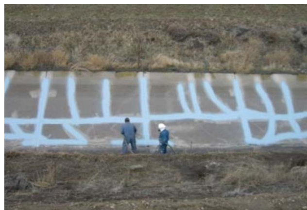
Figure 34: Roza Irrigation District Polyura Application
