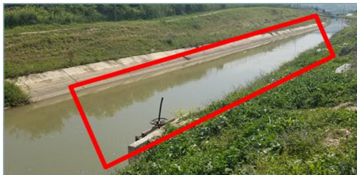
Figure 18: A KAC Reach is Typically Defined as an Uninterrupted Canal Section between Two Check Gates
