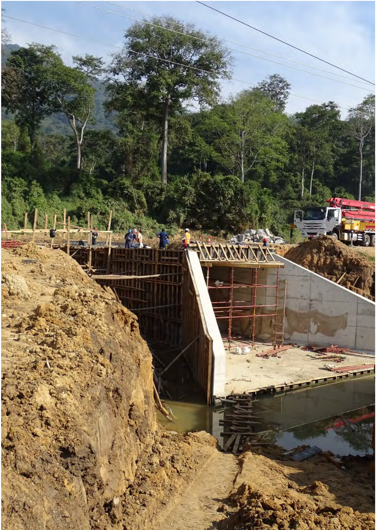
Tanzania's first elephant underpass under construction, July 2020, Mang'ula. Credit: STEP
